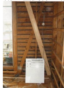
2階洋室筋交取付
