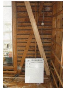
2階洋室筋交取付
